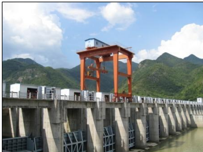
Wuliting Plant, Zhejiang Province Capacity: 42MW
