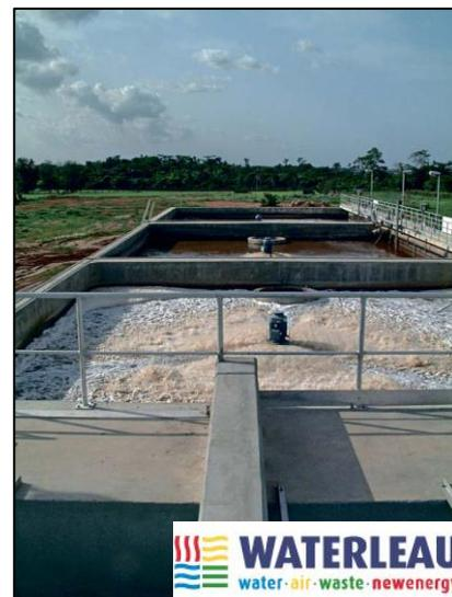
Waterleau's Sequencing Batch Reactor ("SBR") for Heineken in Nigeria.
